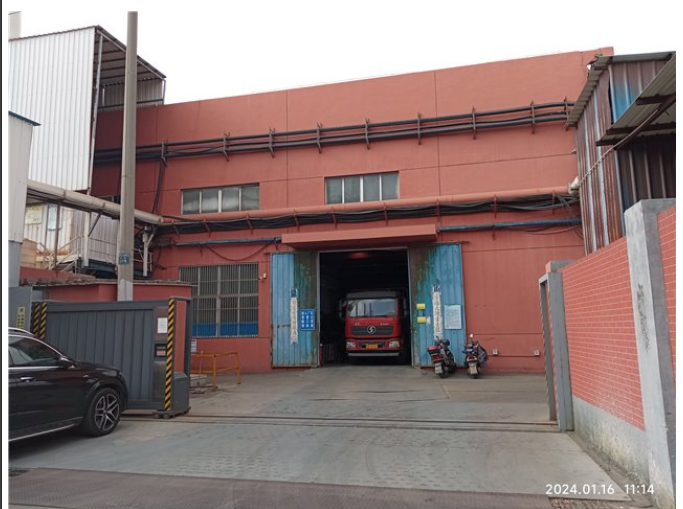
91 - External electroplating factory workshop
