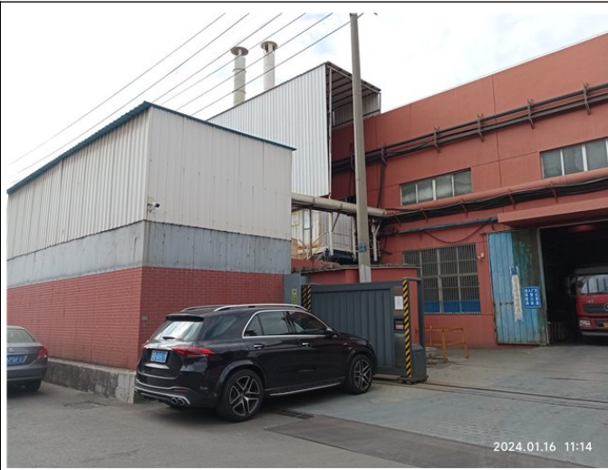
92 - External electroplating factory workshop
