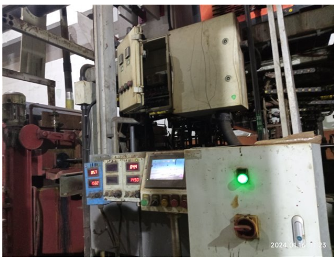
104 - External electroplating factory workshop
