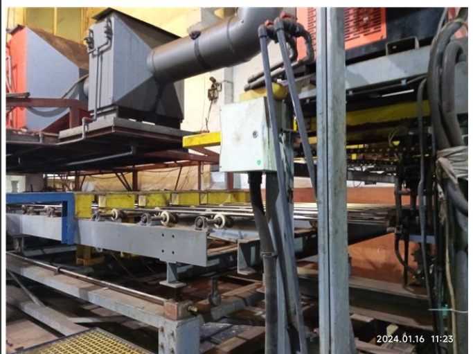
107 - External electroplating factory workshop
